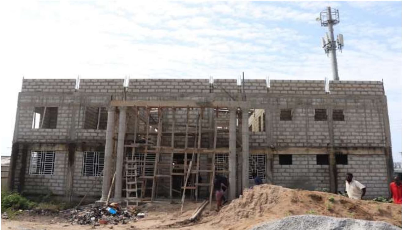
Completion of 30 bed capacity Hospital at Gbegbeyise – 70%
