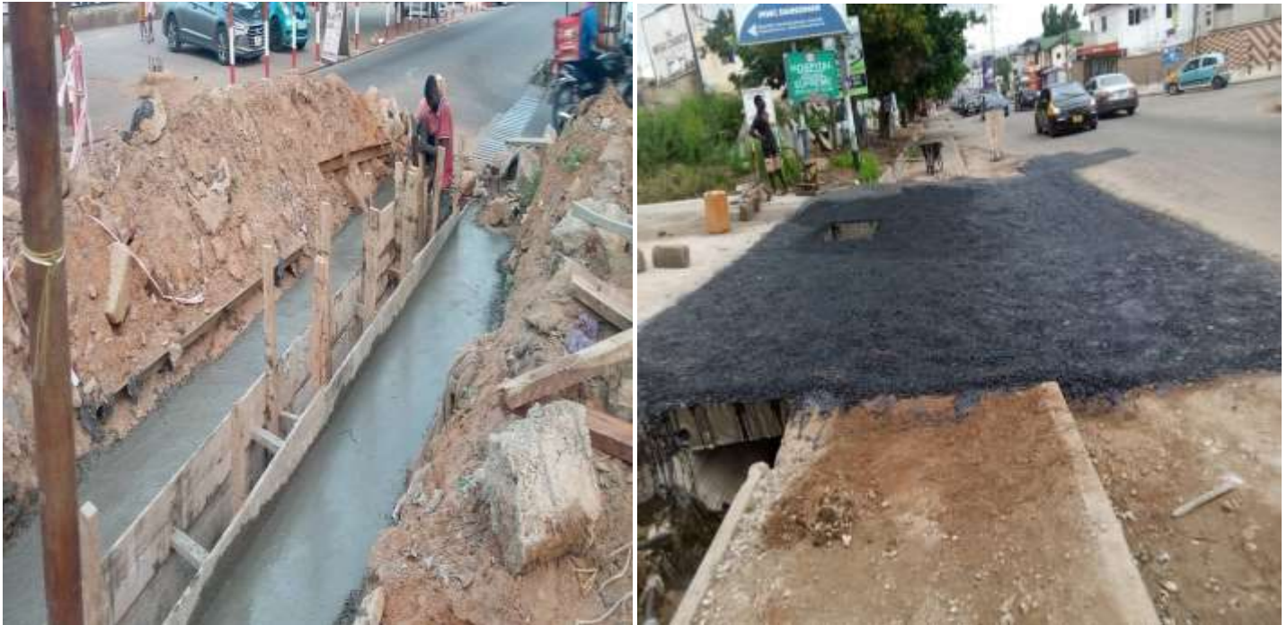
Maintenance Work at 1st Stop and Ave Maria – 100%
