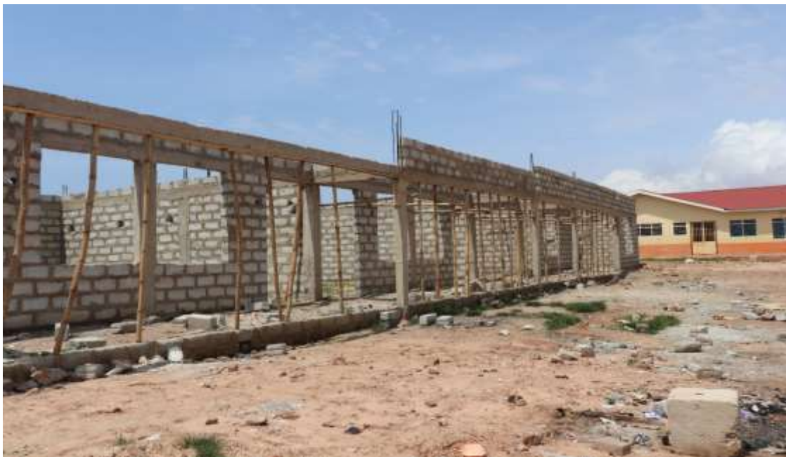
Construction of 1No. 6-Unit Classroom Block @ AME Zion School, Nasarawa. – 55%
