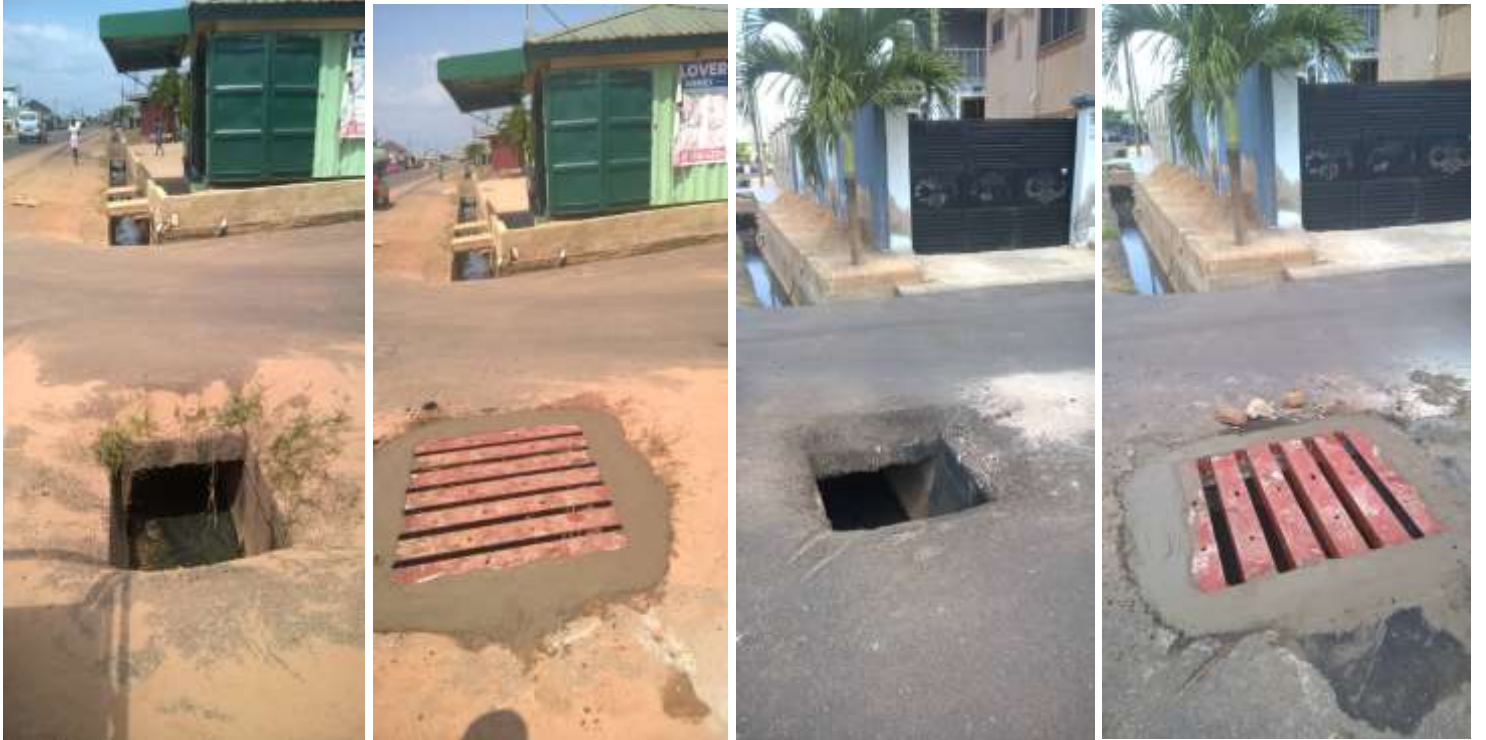
Replacement of Metal Gratings on Selected Roads within the Municipality – 100%
