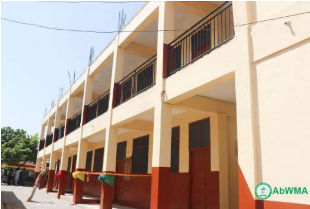
Construction of 1No. 2-Storey 6-Unit Classroom Block @ St. Augustine Ang. – 100% Completed, Handed over and In-use.
